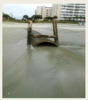
Ocean Outfalls collect storm water regionally, then expel it a quarter-mile offshore via underground pipes. This keeps bacteria-laden storm water out of the "swim zone" and enables us to remove the storm water pipes from the beach
